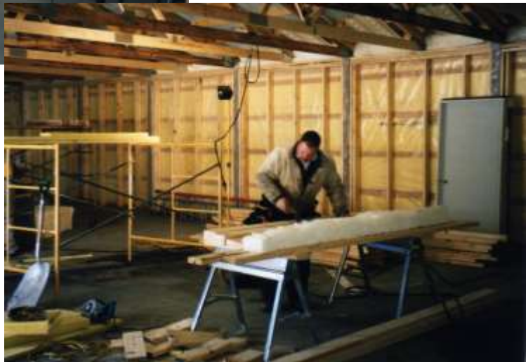
Mr. Shawn Sandmeyer working in February to finish framing the walls and adding supports to the ceiling to remodel the storage area into the Fitness Center.
